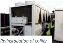
Re-installation of chiller
